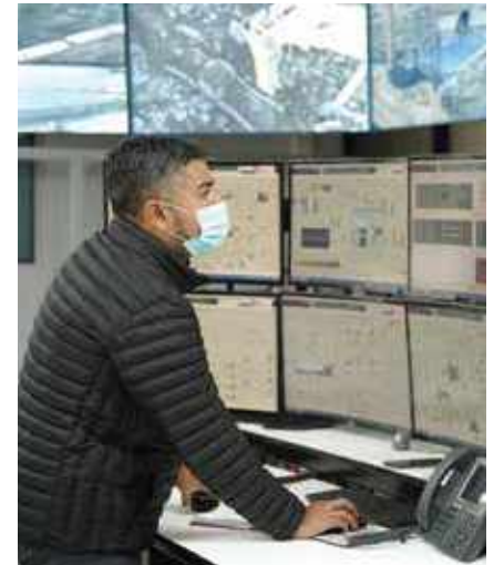
Processing Plant Control Room, Candelaria, Chile
