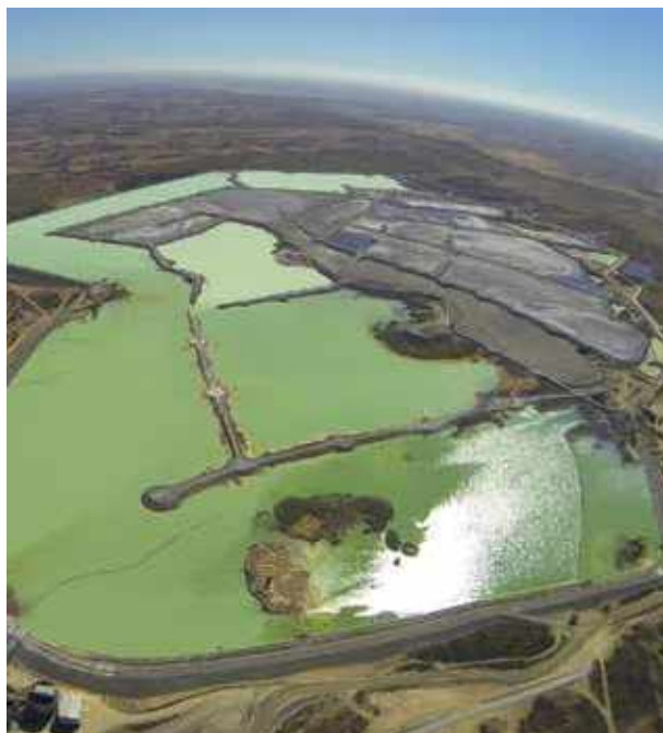
Tailings Facility, Neves-Corvo, Portugal
