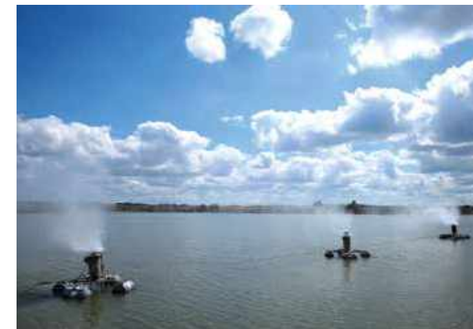
Water Evaporators, Neves-Corvo, Portugal
