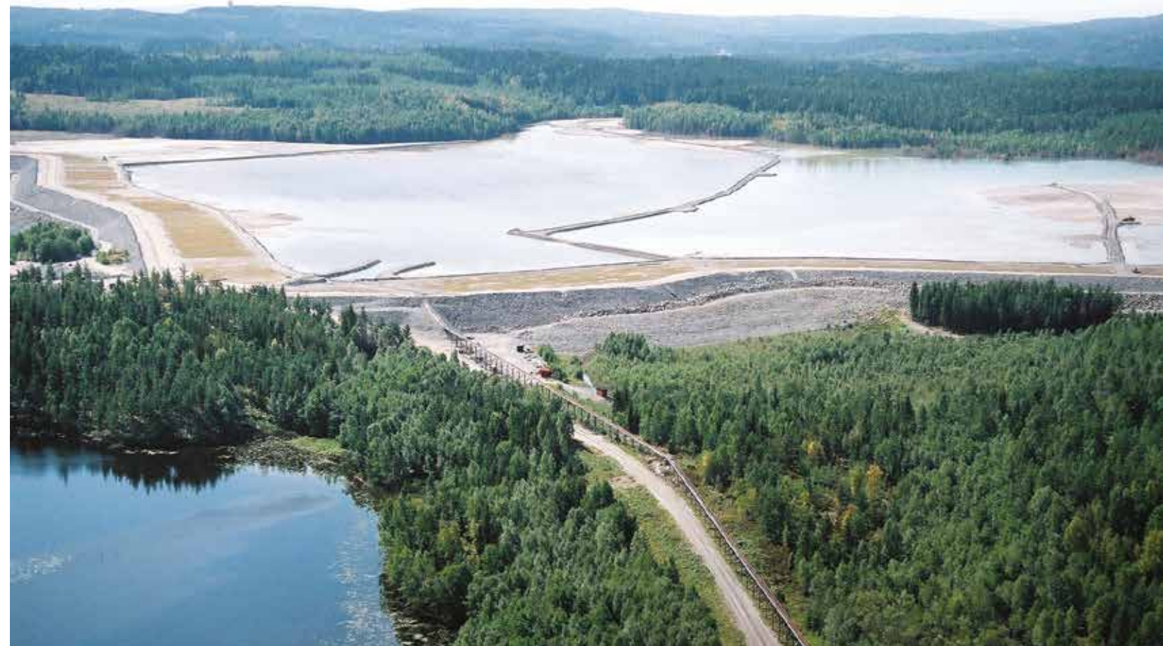
Tailings Facility, Zinkgruvan, Sweden
