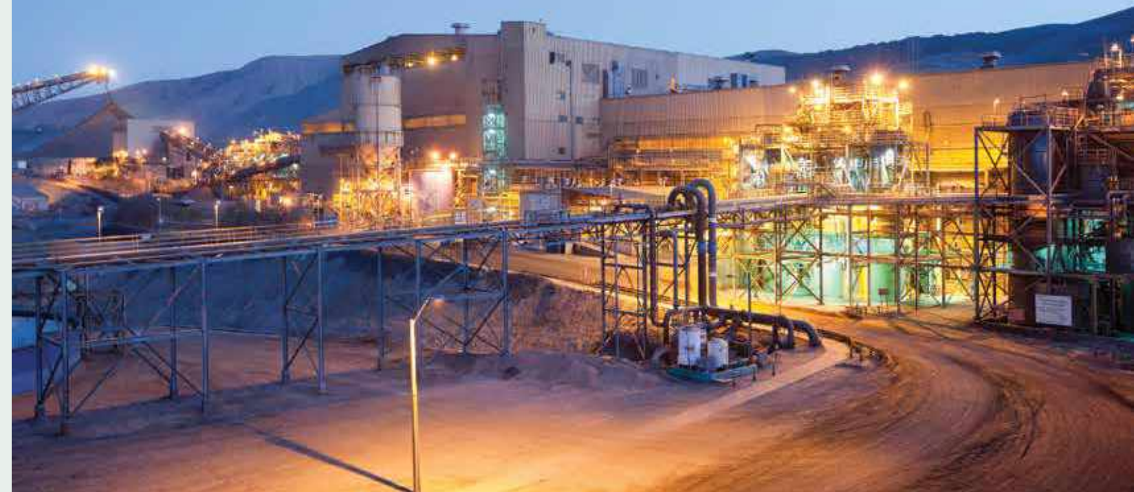
Mill Process Plant, Candelaria, Chile
